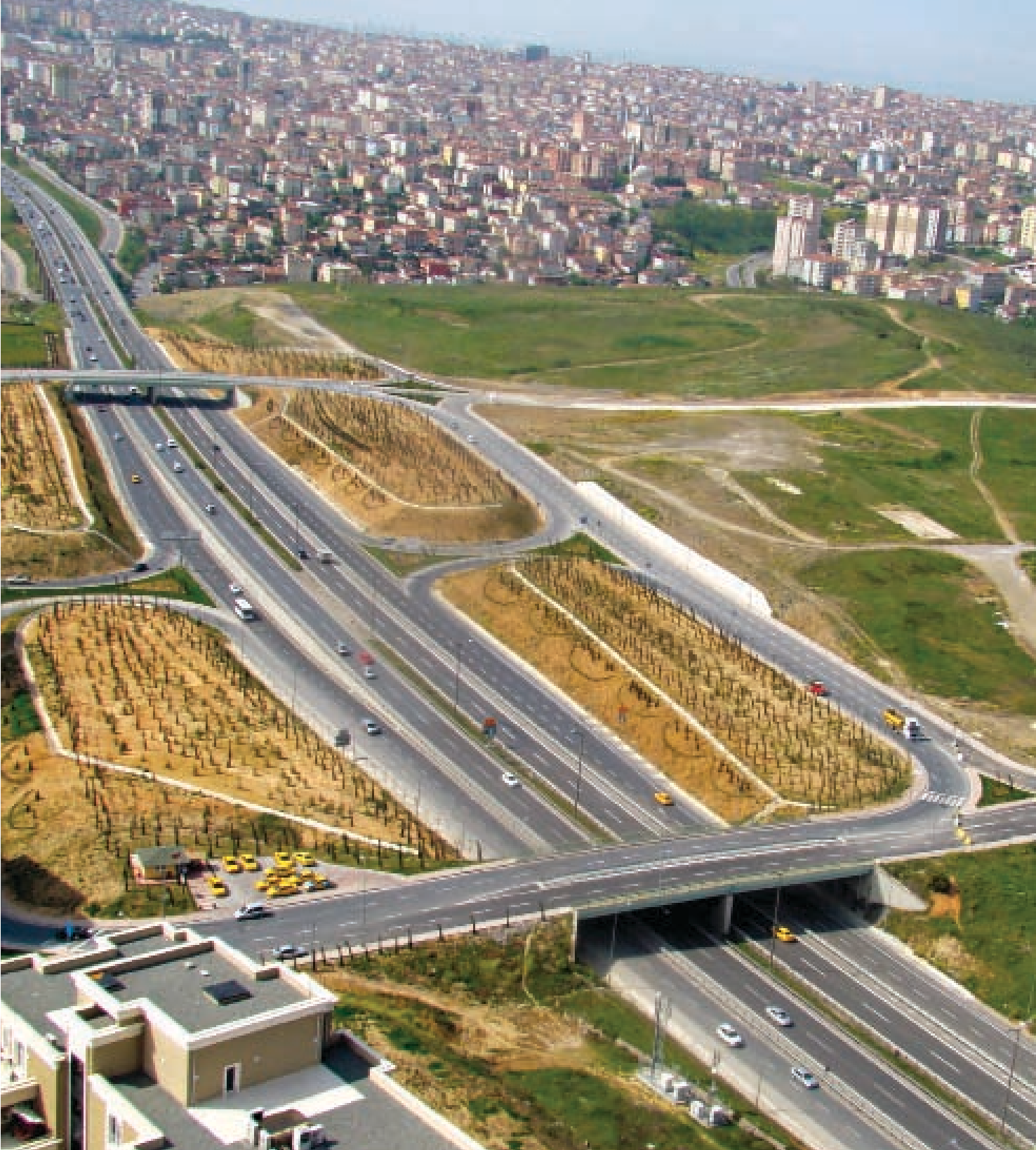
İstanbul-Ataşehir Köprülü Kavşak
